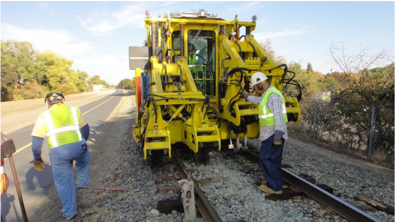
Clem guides Alan in the tamper as Mike F. nips-up a tie
