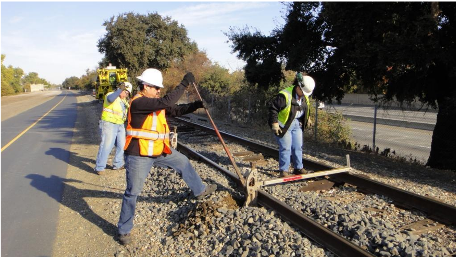
Jose jacks-up the west rail as Heather checks the level
