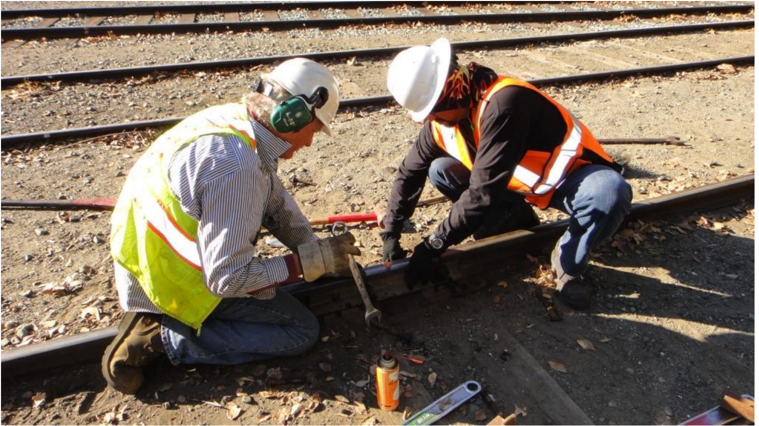
Steve and Jose reassemble the joint
