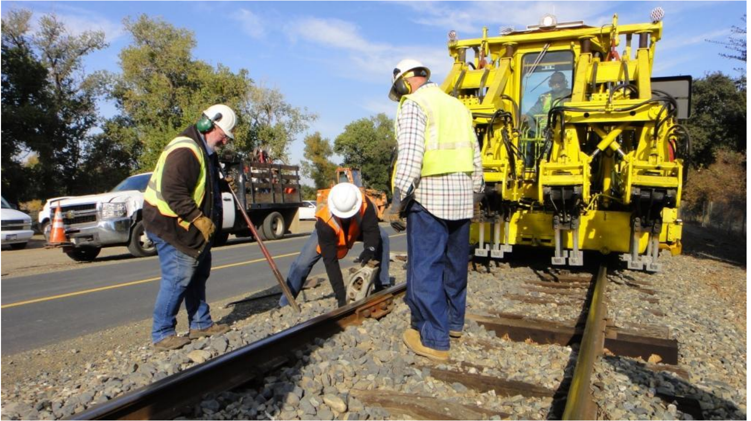
Frank and Jose pull a jack as Alan tamps the rail to the new level guided by Clem
