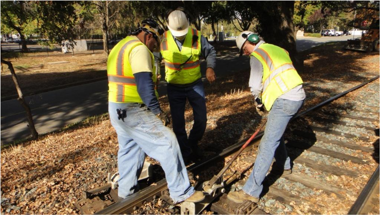
Steve gets the second jack snug in place
