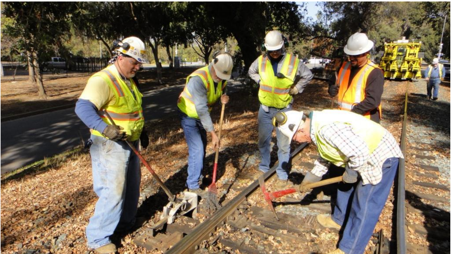
At Switch 14, a jack is placed horizontally against the head-block and the offending tie to shove it slightly south
