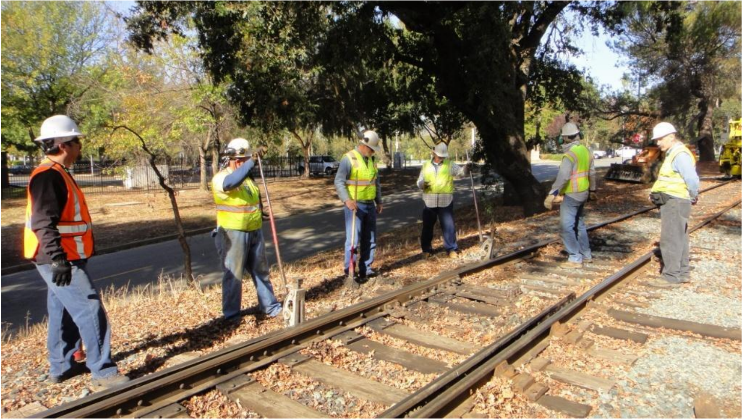
Now jacks are set under the west rail to jack it up so that the west-point will slip into place under the head
