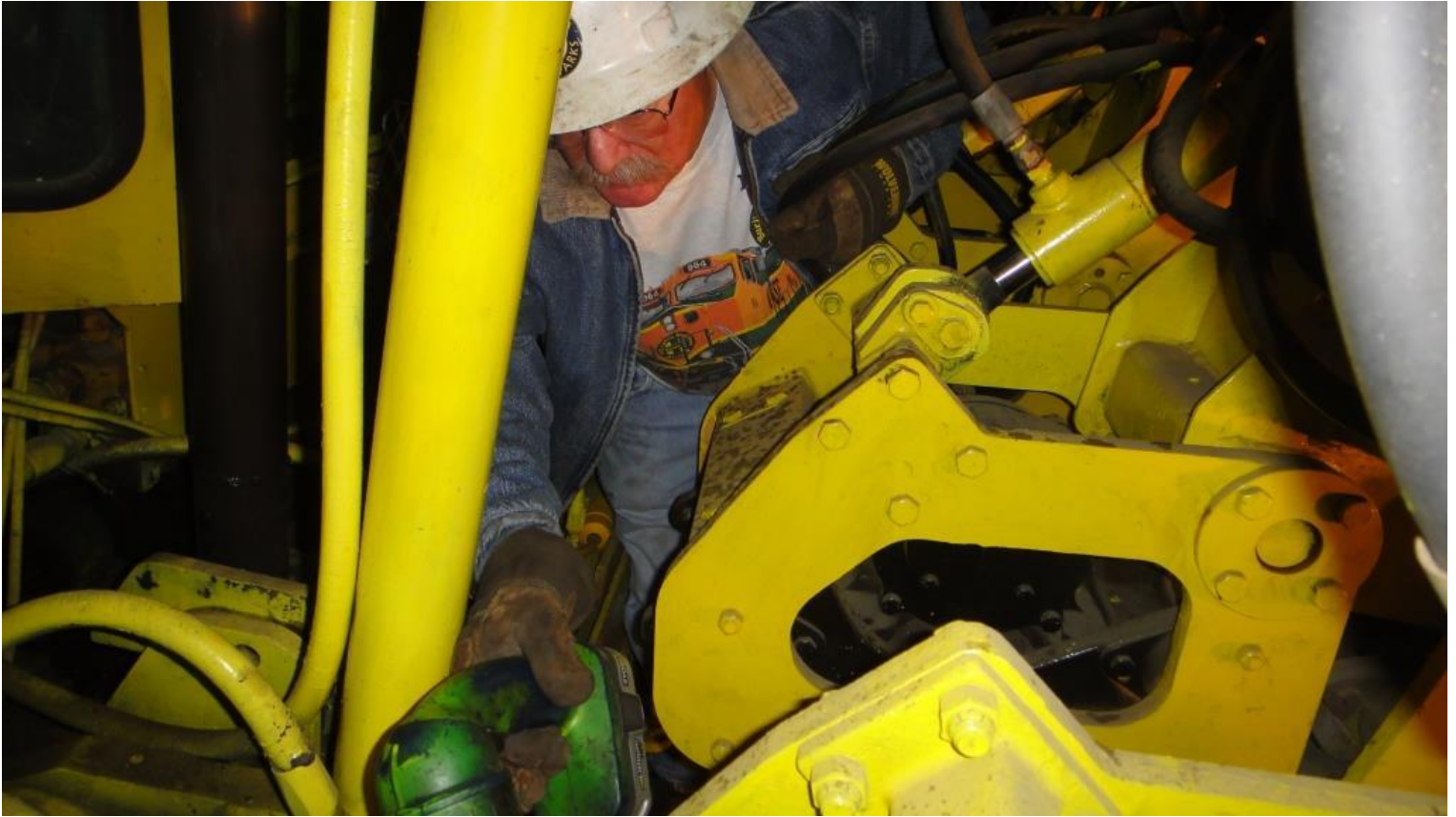
Mike H. climbs into the deep reaches of the tamper to remove cracked work-head buffers
