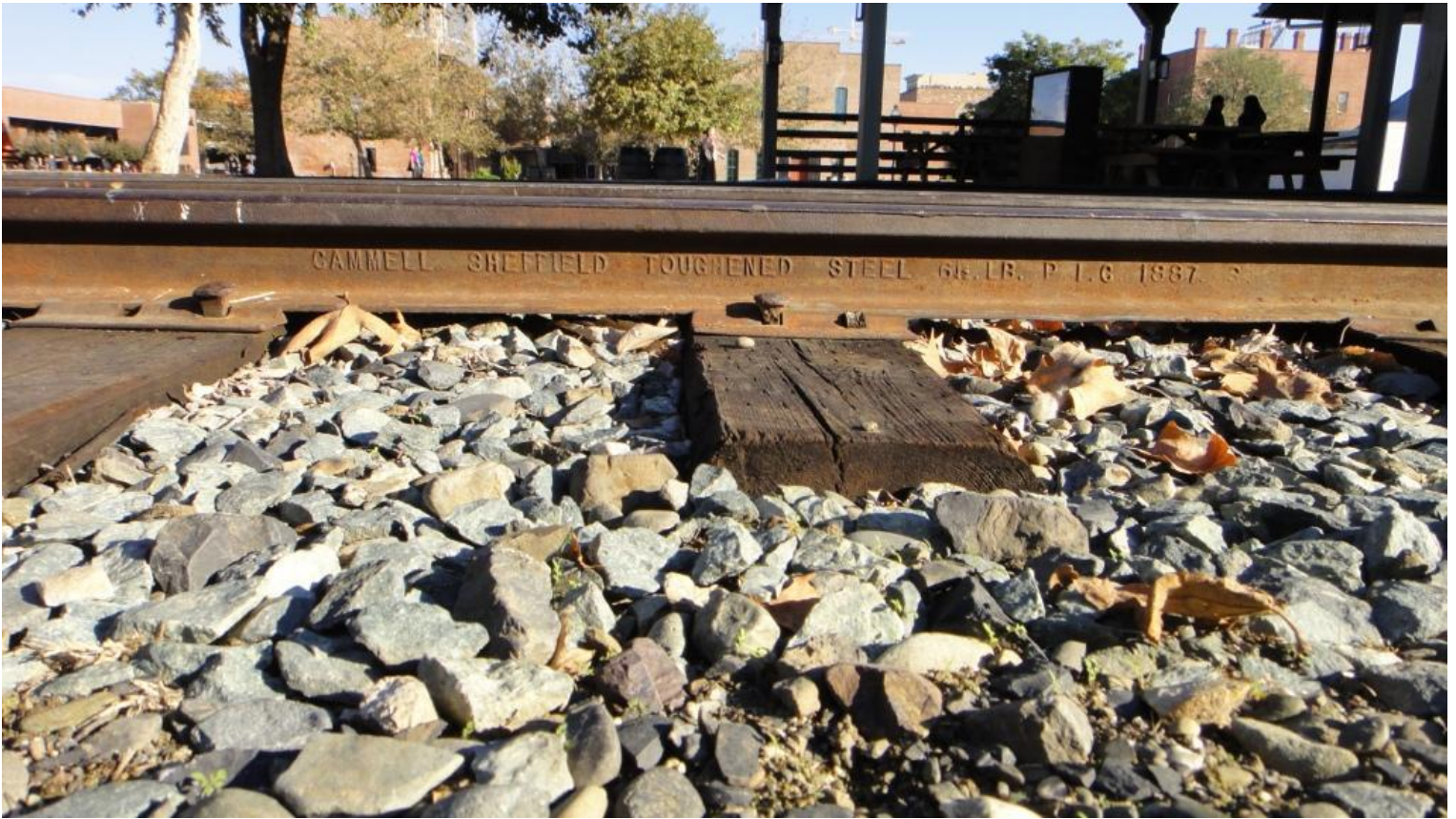
Interpreting our railroad: a stick of 61½ pound rail forged in 1887 by the Charles Cammell & Co, of Cyclops Steel and Iron Works, Sheffield, England
