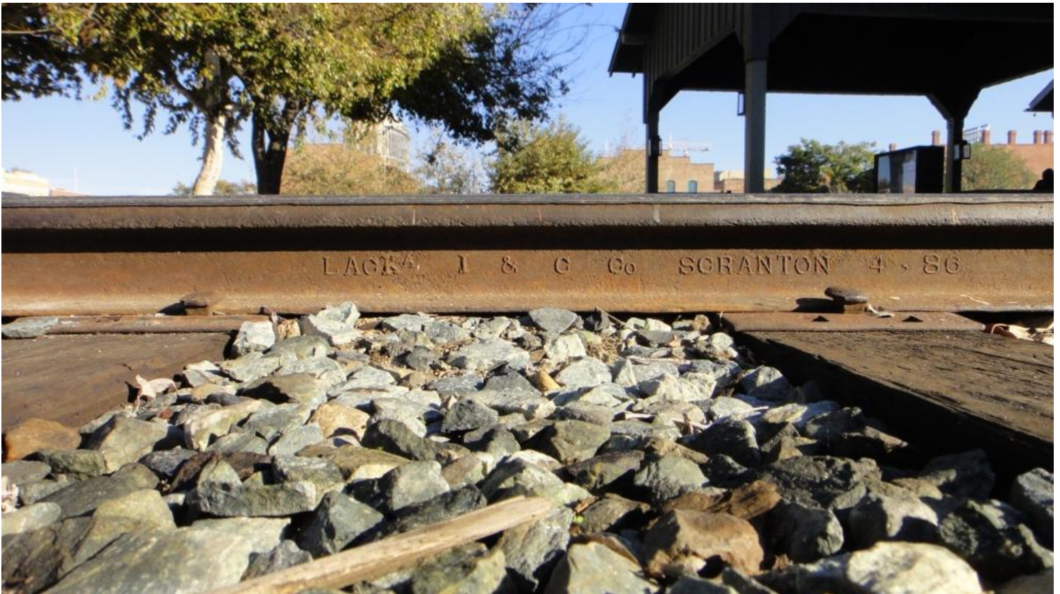
A 129 year old stick of rail forged by the Lackawanna Iron and Coal Company of Scranton, Pennsylvania in April, 1886
