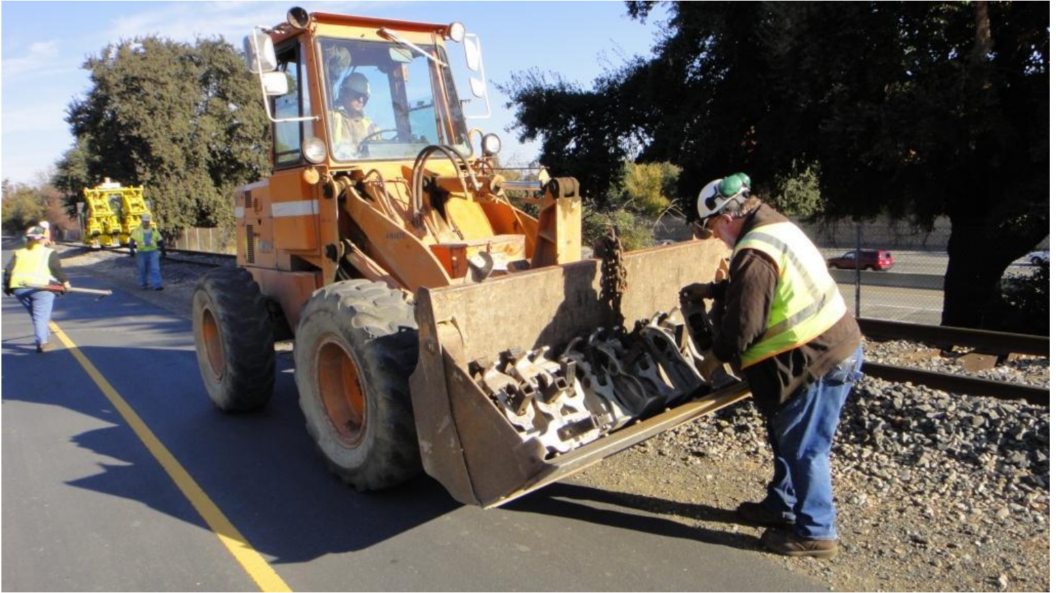
Steve in the loader brings jacks to the work site which Frank deploys
