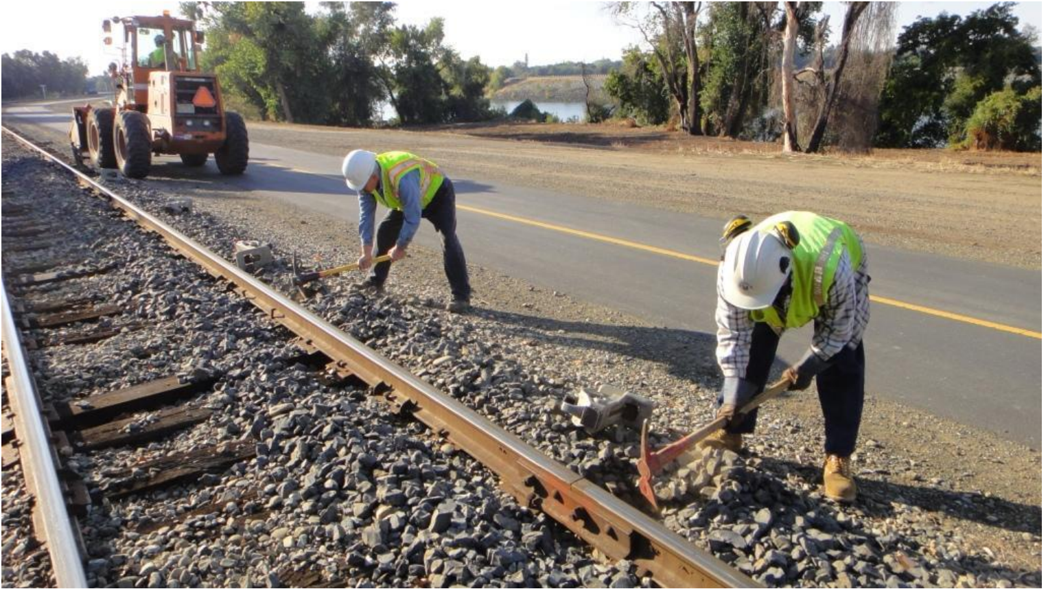
Fred and Clem dig-out the ballast from under the base of the rail so jacks can be set
