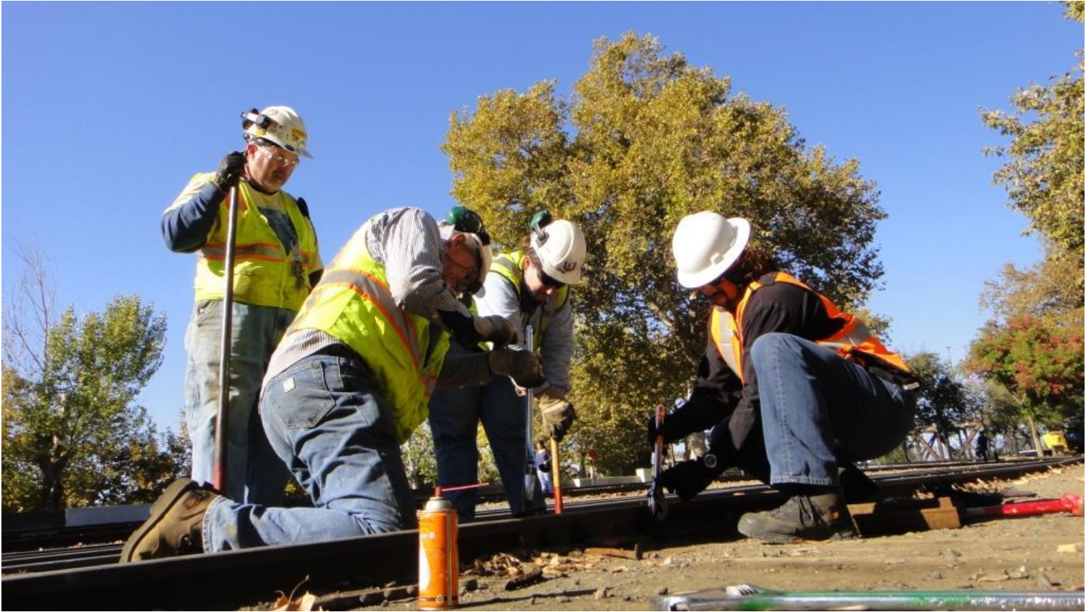
Back in Old Sacramento, Mike F., Steve, Heather, and Jose take apart the joint on the CPPS Track with the cracked joint-bar
